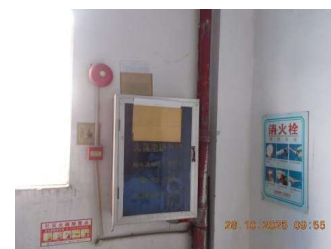
Fire alarm and fire hydrant.JPG
